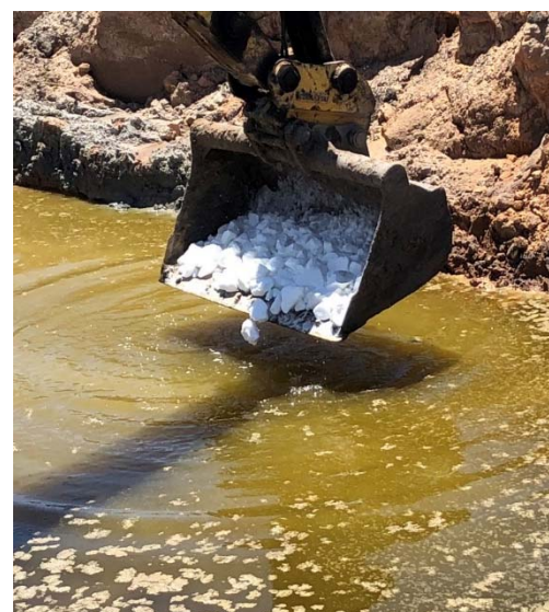
Photo 6: Addition of chemical oxidant to saturated soils within open excavation to enhance biodegradation
